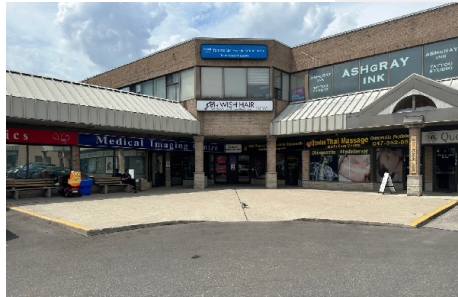
398 Steeles Avenue West, Vaughan
