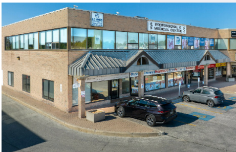
390 Steeles Avenue West, Vaughan
