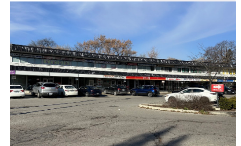
2428 Islington Avenue, Toronto
