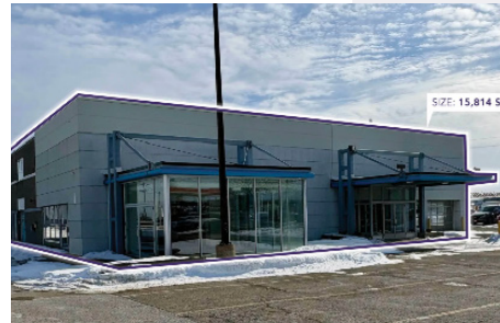
8046 Dixie Road, Car Dealership, Brampton
