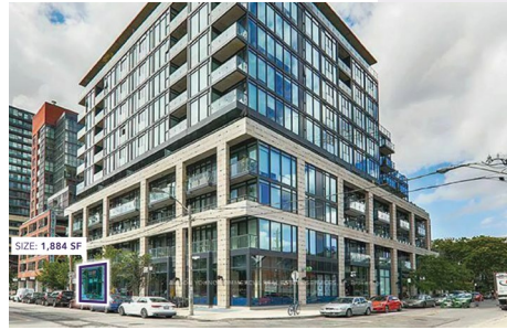
66 Sudbury Street, Toronto
