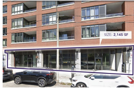
80 Sudbury Street, Toronto
