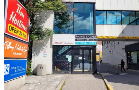
550 St. Clair Avenue West, Units 204 & 209, Toronto
