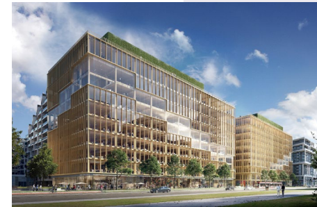
251 Queens Quay East, Toronto
