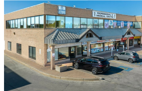
390 Steeles Avenue West, Vaughan
