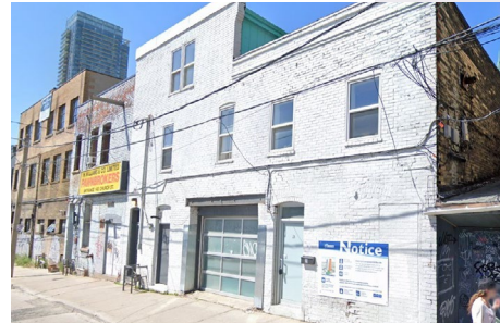
20 Dalhousie Street, Toronto
