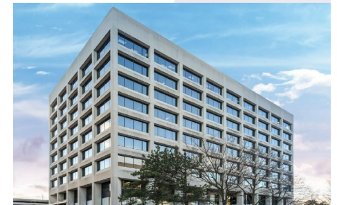
225 Duncan Mill Road, Toronto
