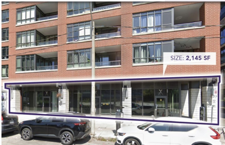
80 Sudbury Street, Toronto
