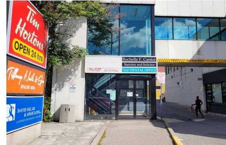
550 St. Clair Avenue West, Units 204 & 209, Toronto
