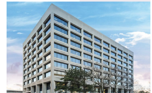
225 Duncan Mill Road, Toronto
