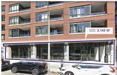
80 Sudbury Street, Toronto
