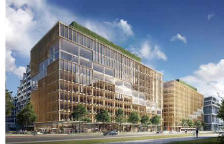
251 Queens Quay East, Toronto
