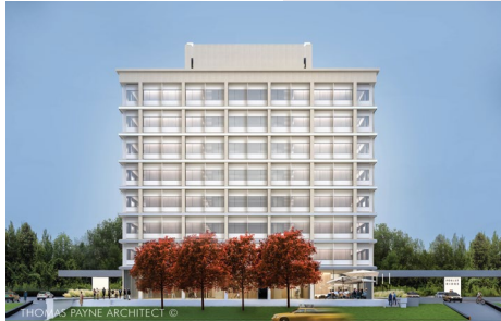
240 Duncan Mill Road, Toronto
