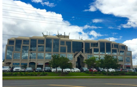
1600 Steeles Avenue West, Vaughan
