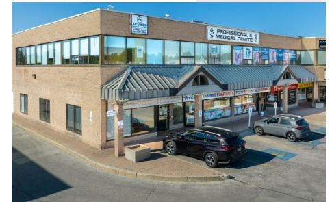
390 Steeles Avenue West, Vaughan
