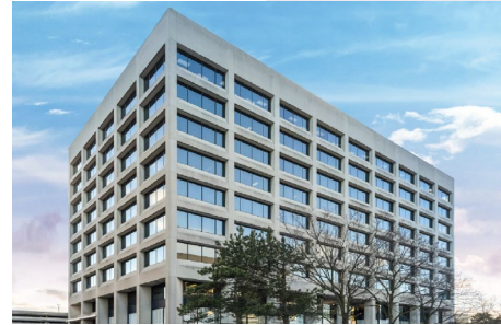
225 Duncan Mill Road, Toronto
