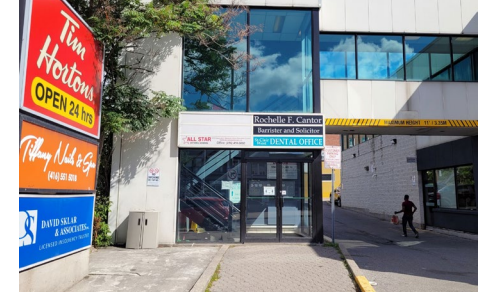
550 St. Clair Avenue West, Units 204 & 209, Toronto
