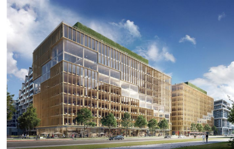
251 Queens Quay East, Toronto
