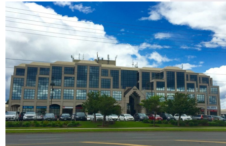
1600 Steeles Avenue West, Vaughan
