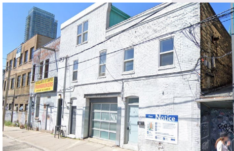
20 Dalhousie Street, Toronto
