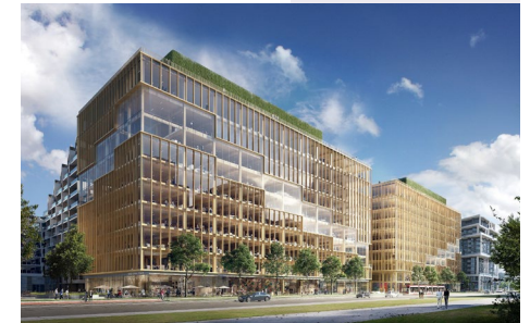
251 Queens Quay East, Toronto
