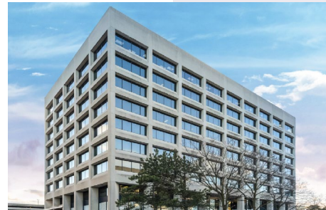
225 Duncan Mill Road, Toronto
