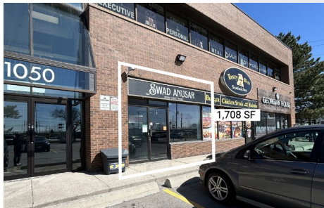
1048 Finch Avenue West, Toronto
