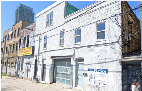
20 Dalhousie Street, Toronto
