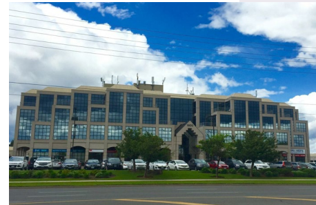
1600 Steeles Avenue West, Vaughan
