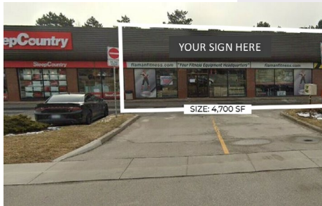
3300 Fairview Street, Unit 2, Burlington
