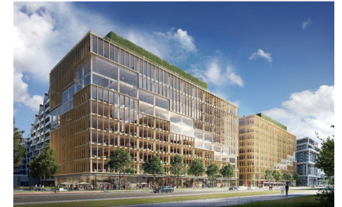
251 Queens Quay East, Toronto
