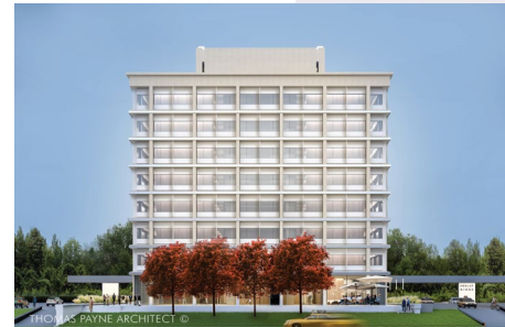
240 Duncan Mill Road, Toronto
