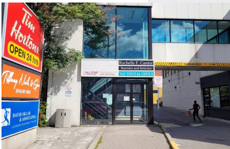
550 St. Clair Avenue West, Units 204 & 209, Toronto
