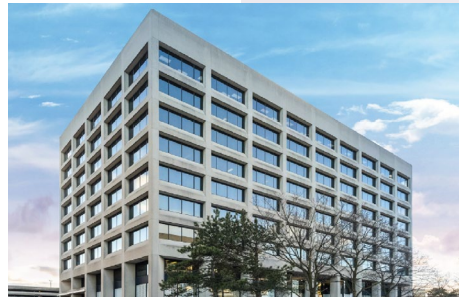
225 Duncan Mill Road, Toronto
