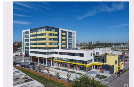
1275 Finch Avenue West, Unit 210-214, Toronto
