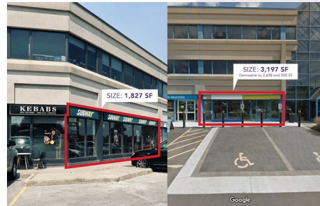
2180 Steeles Avenue West, Vaughan
