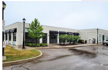
6 Thompson Crescent, Unit 2-5, Erin
