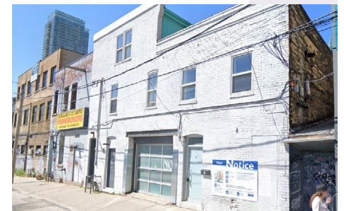
20 Dalhousie Street, Toronto
