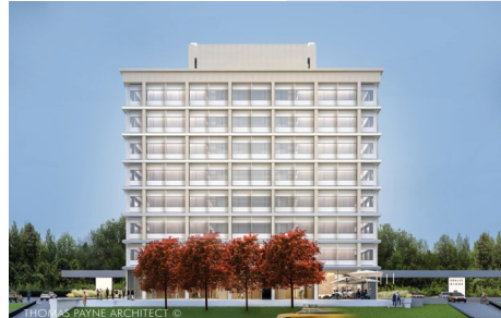
240 Duncan Mill Road, Toronto
