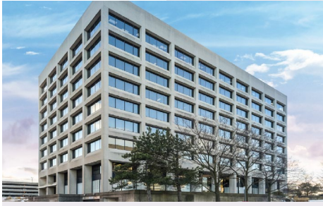
225 Duncan Mill Road, Toronto
