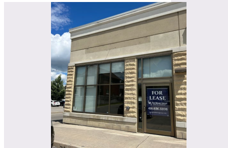
1 Warren Road, Unit 107, Oshawa, Oshawa
