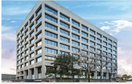
225 Duncan Mill Road, Toronto
