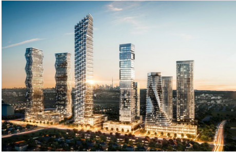
Burnhamthorpe Road West & Confederation Parkway, Mississauga
