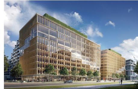
251 Queens Quay East, Toronto
