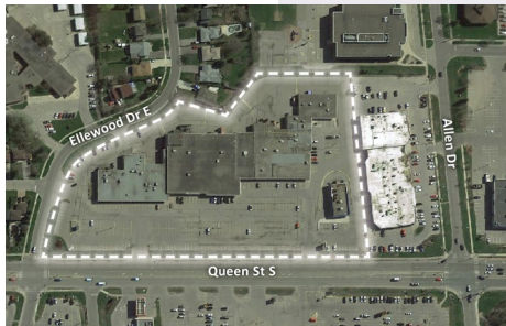
301 Queen Street South, Bolton
