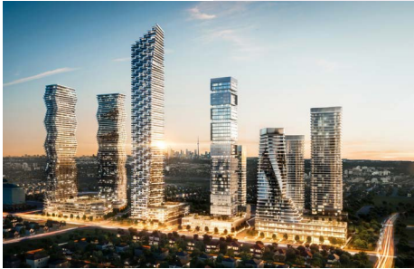
Burnhamthorpe Road West & Confederation Parkway, Mississauga
